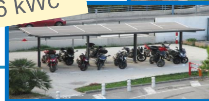
Station de recharge & panneaux photovoltaïques
